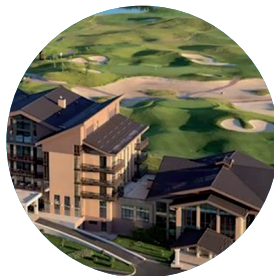
Superior Golf & SPA Resort / Ukraine Pump station & irrigation system installation
